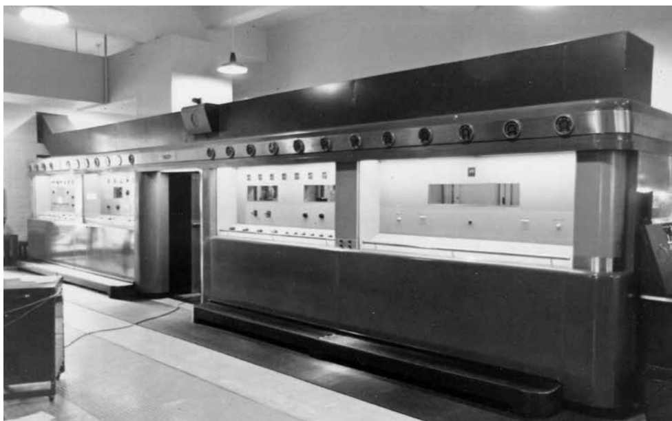
100 kilowatt General Electric -short wave transmitter in Okinawa, 1968.
